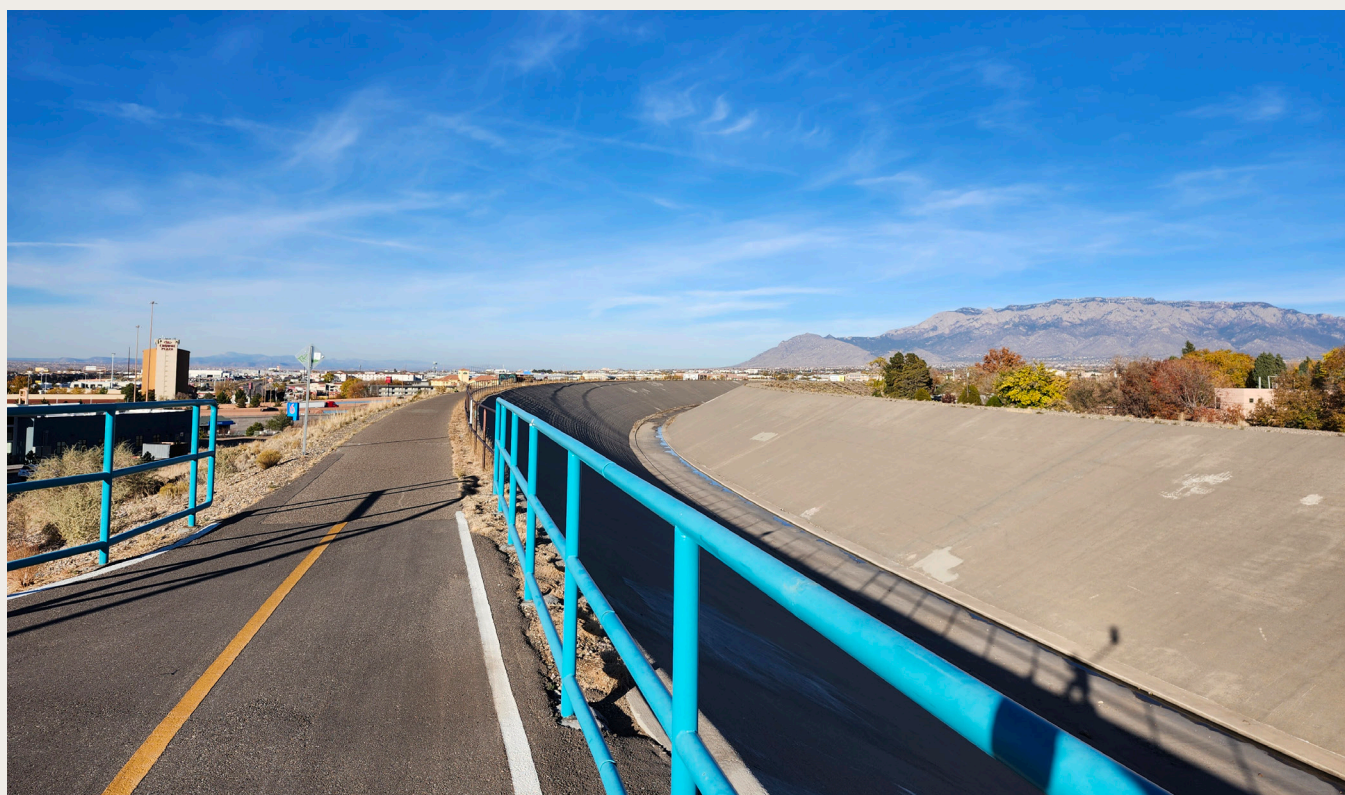
Albuquerque arroyo. Dry most of the time, the system accepts short deluges of storm water.
